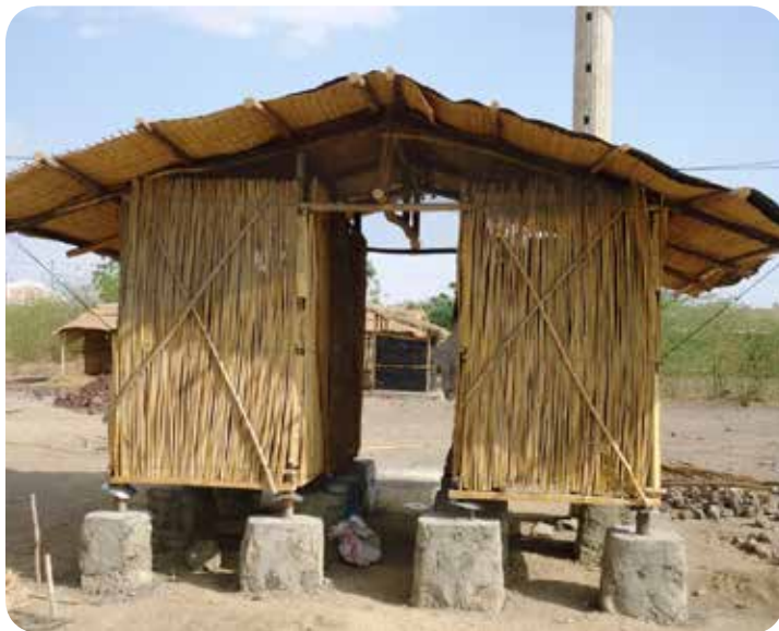
Ventilated onion storage structure, showing rat guards [Tool 75] and shade cover, designed by Mekbib Heitegebrile Seife - PEF Graduate, Ethiopia, 2012 - Photo: Lisa Kitinoja
