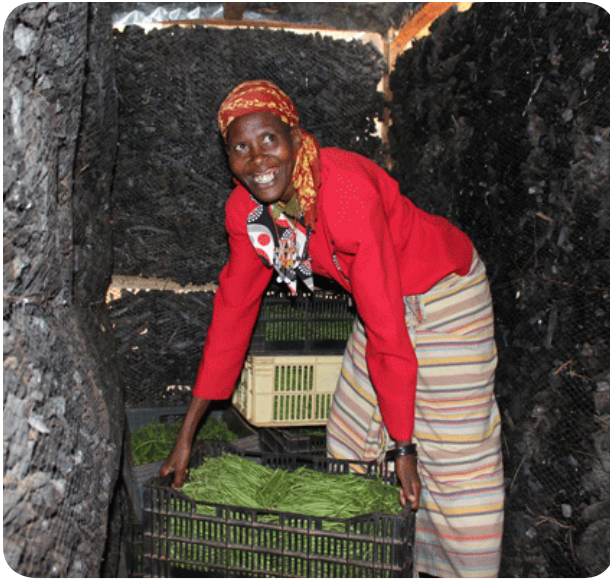
Mary Gatumitha, a member of the Bindii Farmers Group, stores their contract French green beans in their evaporative charcoal cooler, Biolo, Kenya - Photo: Pauline Kairu, permission requested
