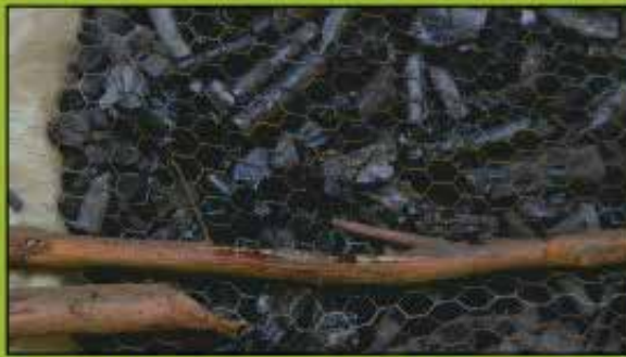
The open walls are made of mesh wire packed with charcoal.
