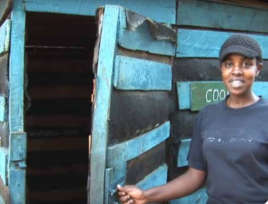
Virginia Wango explains an evaporative charcoal cooler for storing green beans - Photo: YouTube/Green Shots [bit.ly/2MeJRaXj] Mitja Mithans
