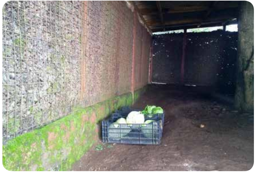
Produce cooled in a 30 square meter charcoal cooler in Tanzania [ bit.ly/2P7KqBp ]; solar panels run a water pump to moisten the walls and the water dripping through is collected in gutters under the walls to be recirculated - Photo: © Marc van der Sterren
