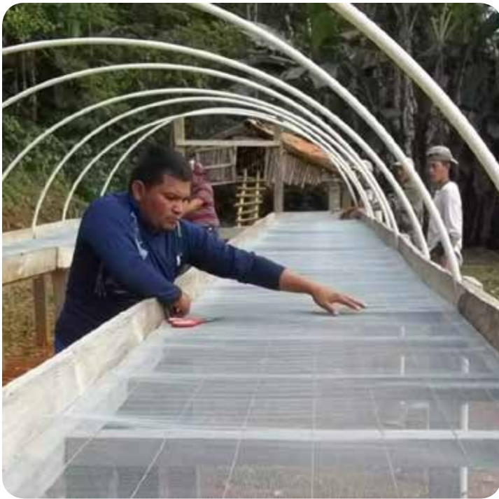
Stretching screening on drying frames for a high tunnel solar grain dryer - Photo: Fintrac
