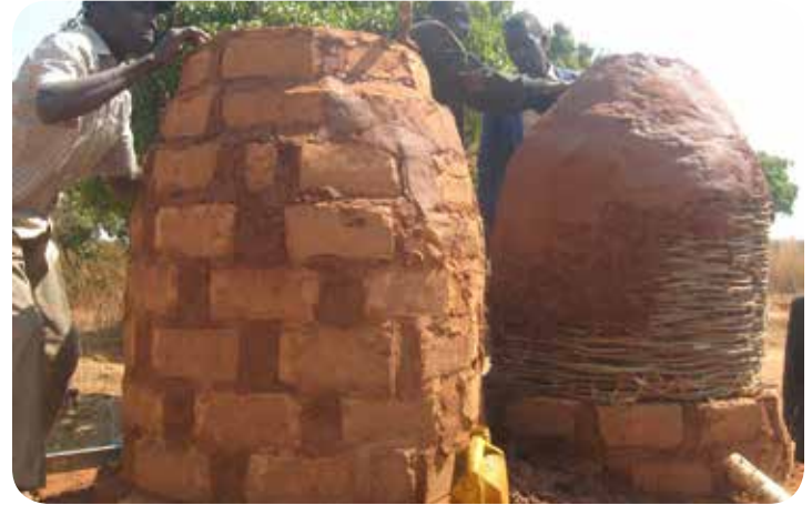
Mud silos under construction in Ghana - Photographer: Pertina Nyamukondiwa/USAid
