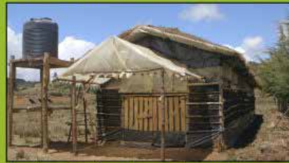
The charcoal is always kept wet by water from a tank. Water evaporates from the charcoal which takes heat from inside the store. The store is therefore kept very cold.
