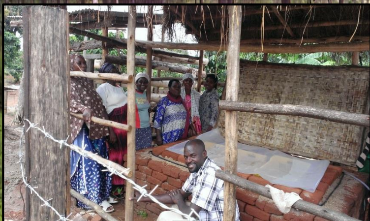
Wilberforce Myumba with women farmers and completed Zero Energy Cooling Chamber (ZECC)
