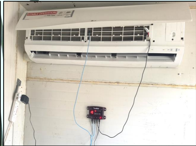
CoolBot unit in the cold room
