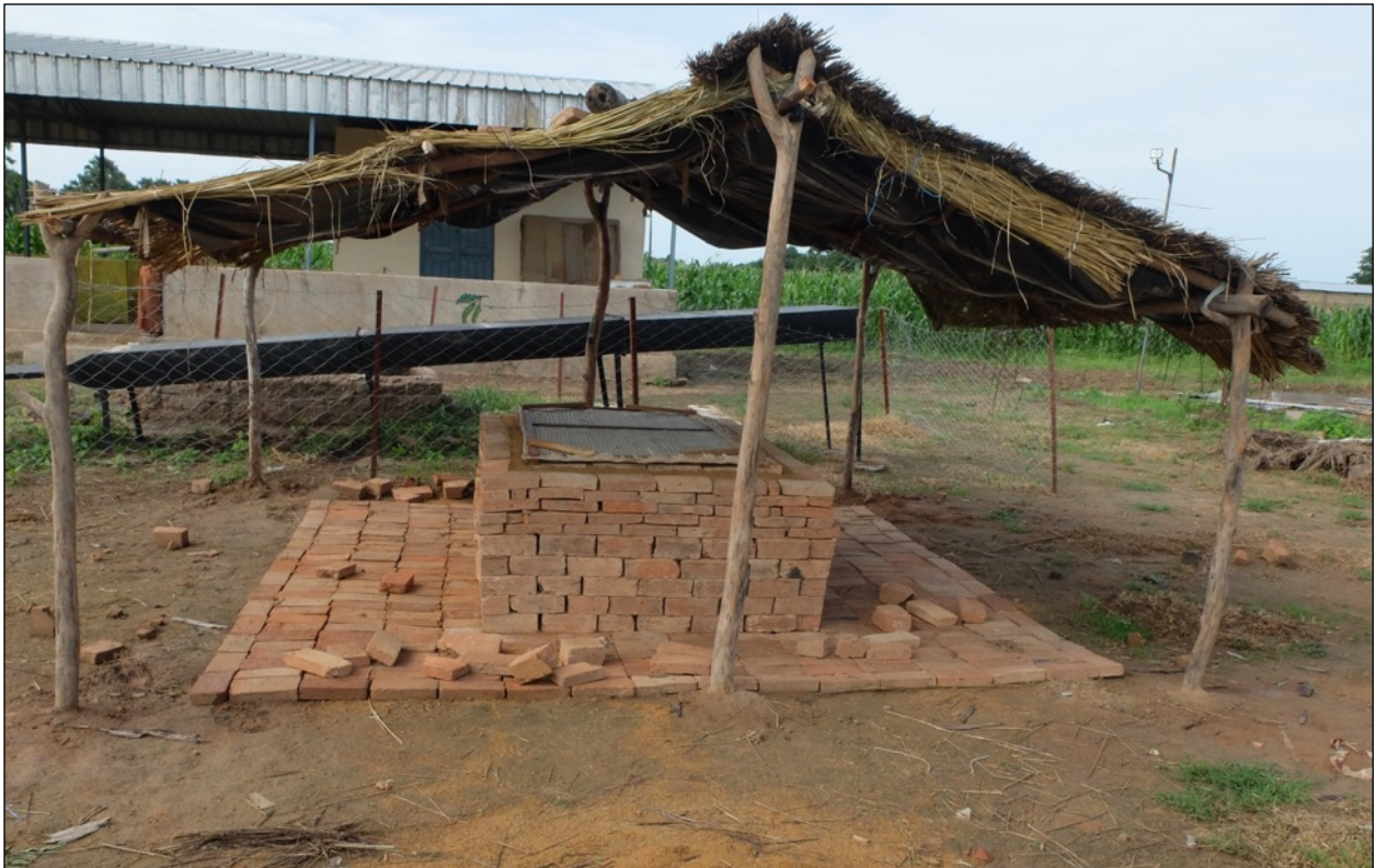
An evaporative cooling chamber (ECC) under a shade cover made from wood, straw, and plastic
