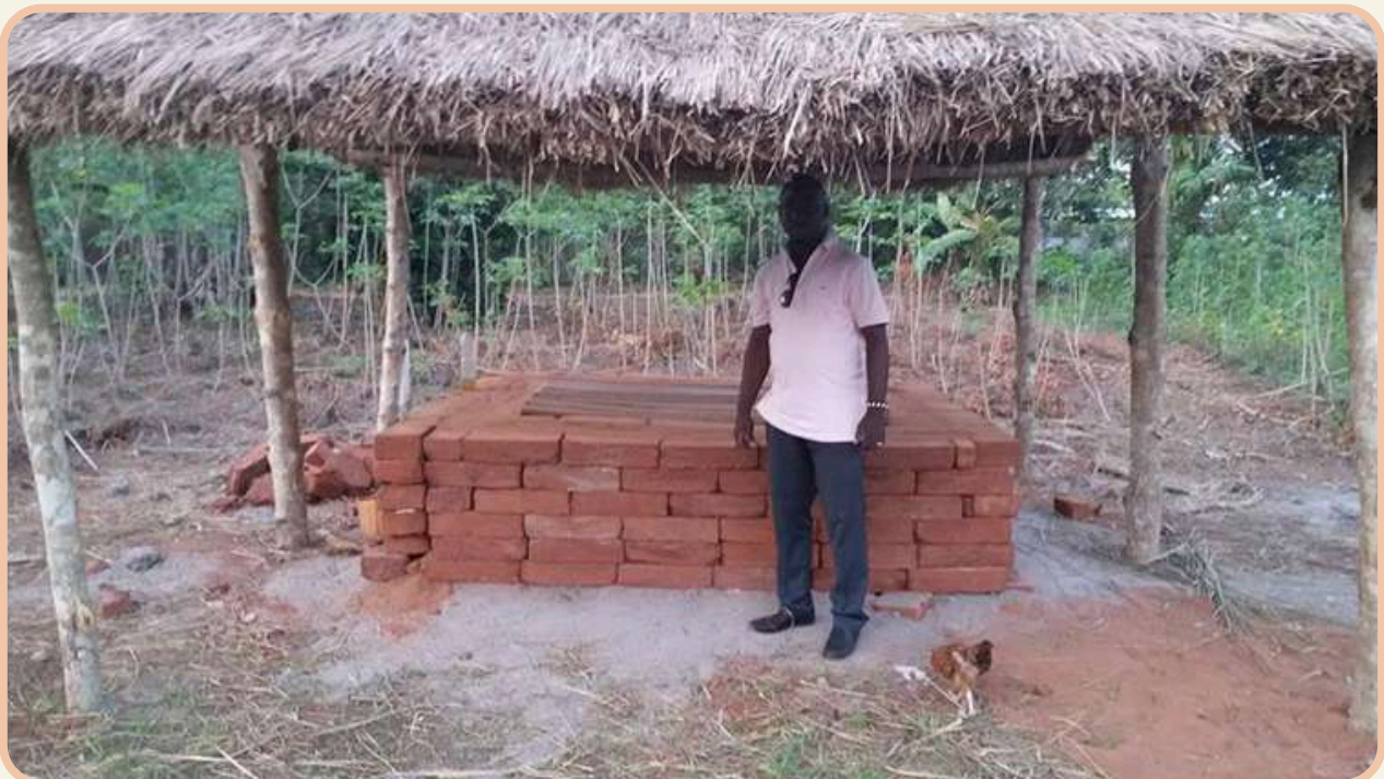
Photo of a Zero Energy Cool Chamber (ZECC) being constructed on a farm in Benin by Guy Kodjogbe
